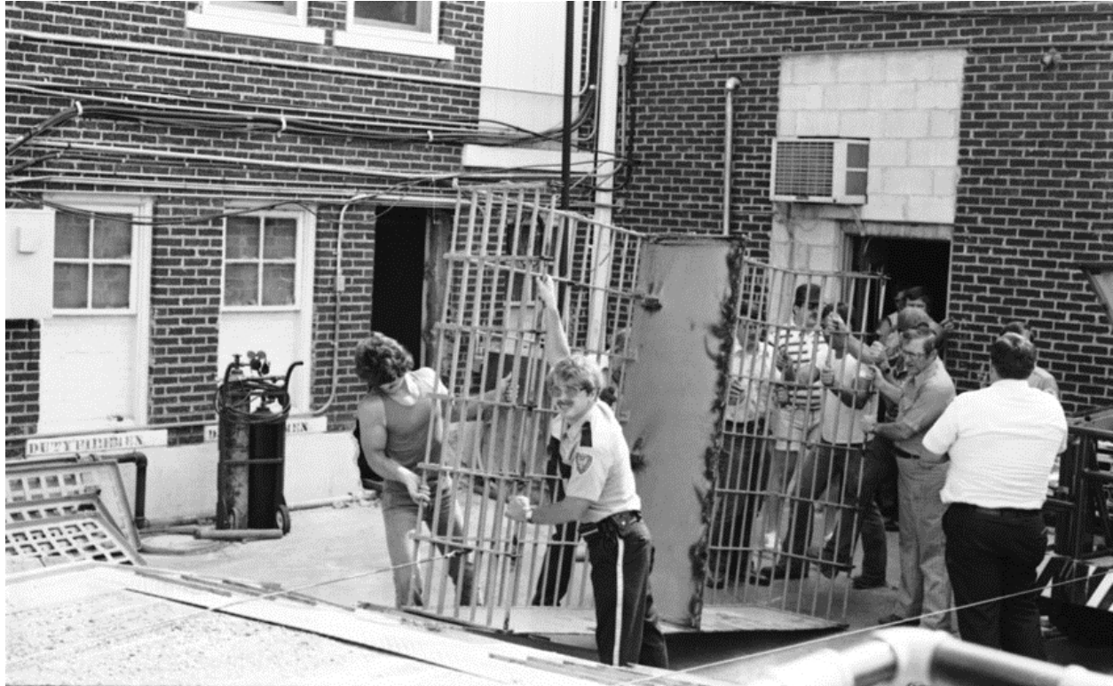
1894 City Jail Cells Being Removed from the Rogers Police Department in 1979 Rogers City Hall, 214 West Elm Street Photo Courtesy Dennis Patton
